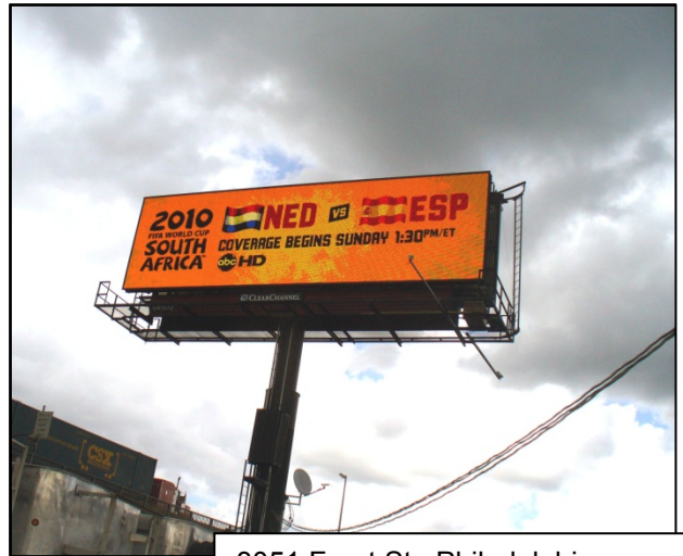
3051 Front St., Philadelphia Off-premise LED sign
