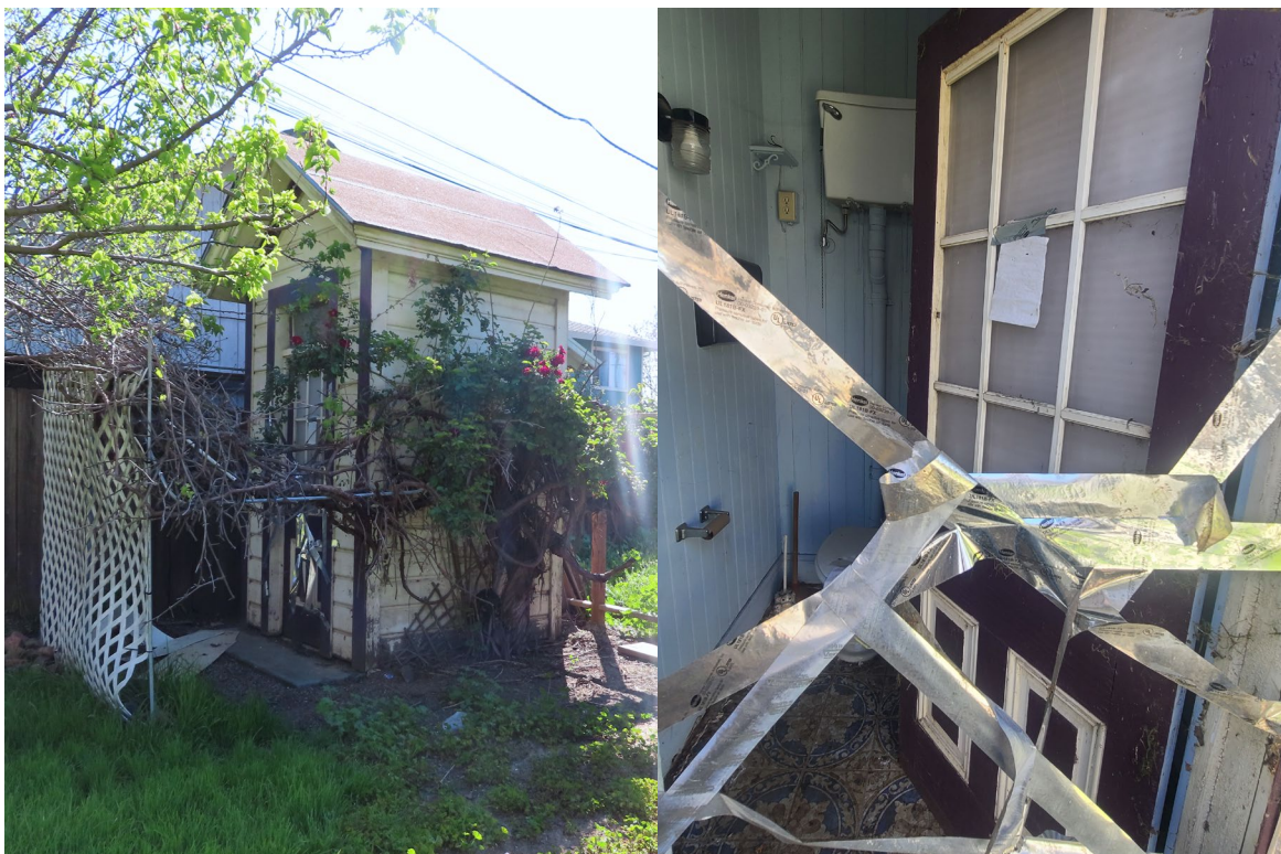
Photograph 2. The Former Greenhouse building that was remodeled into a bathroom in the early-to-mid 20th century, view looking southeast (IMG_1082 and IMG_1140).
