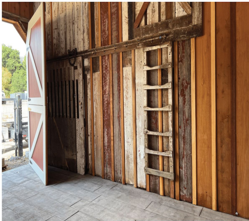
View toward location for group A (ladder to be removed / relocated)
