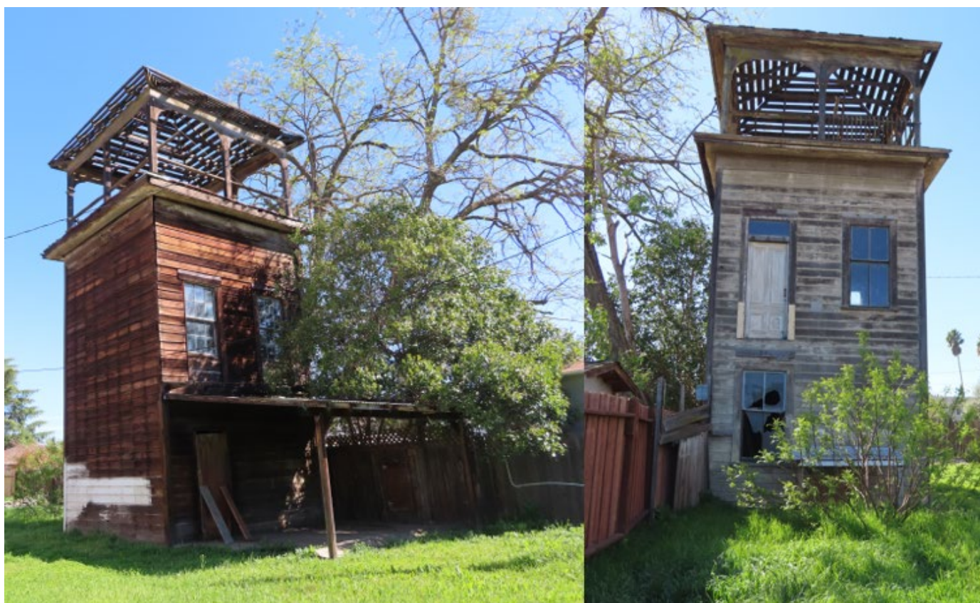
Photograph 1. The west and south elevations (left) of the Tank House, view looking northeast, and north elevation (right), view looking south (IMG_1087 and IMG_1097).
