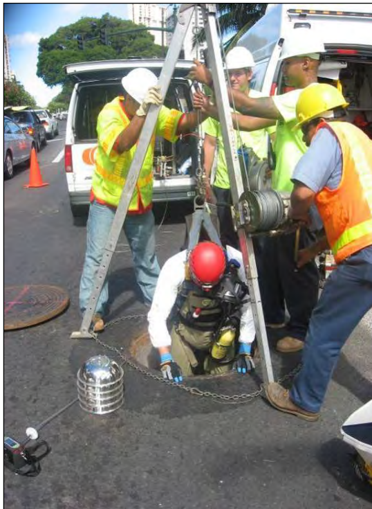
Photo 1. Confined Space Entry
