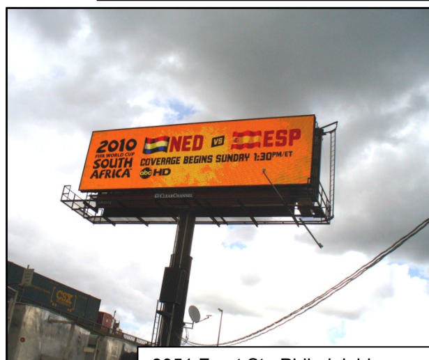
3051 Front St., Philadelphia Off-premise LED sign
